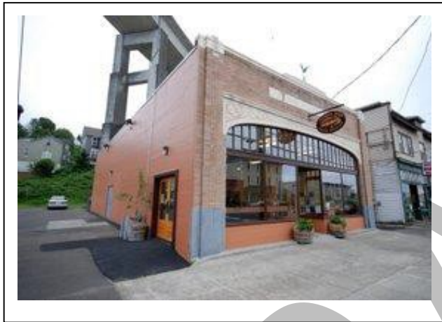
Figure 14.____- _: Non-Industrial Building, Flat Roof Behind Parapet Wall
