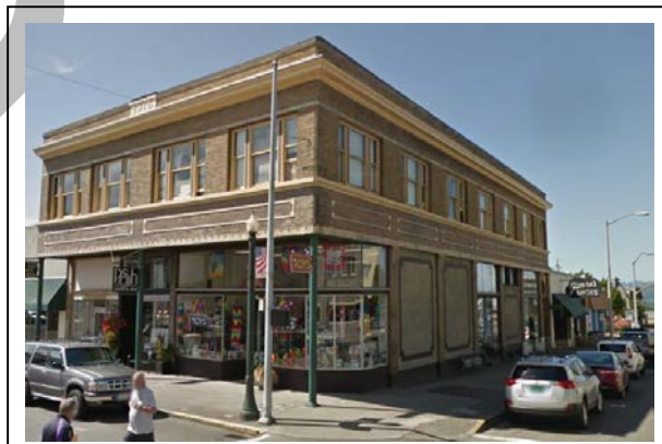
Figure 14.____-__: Base, Middle & Top of Building
