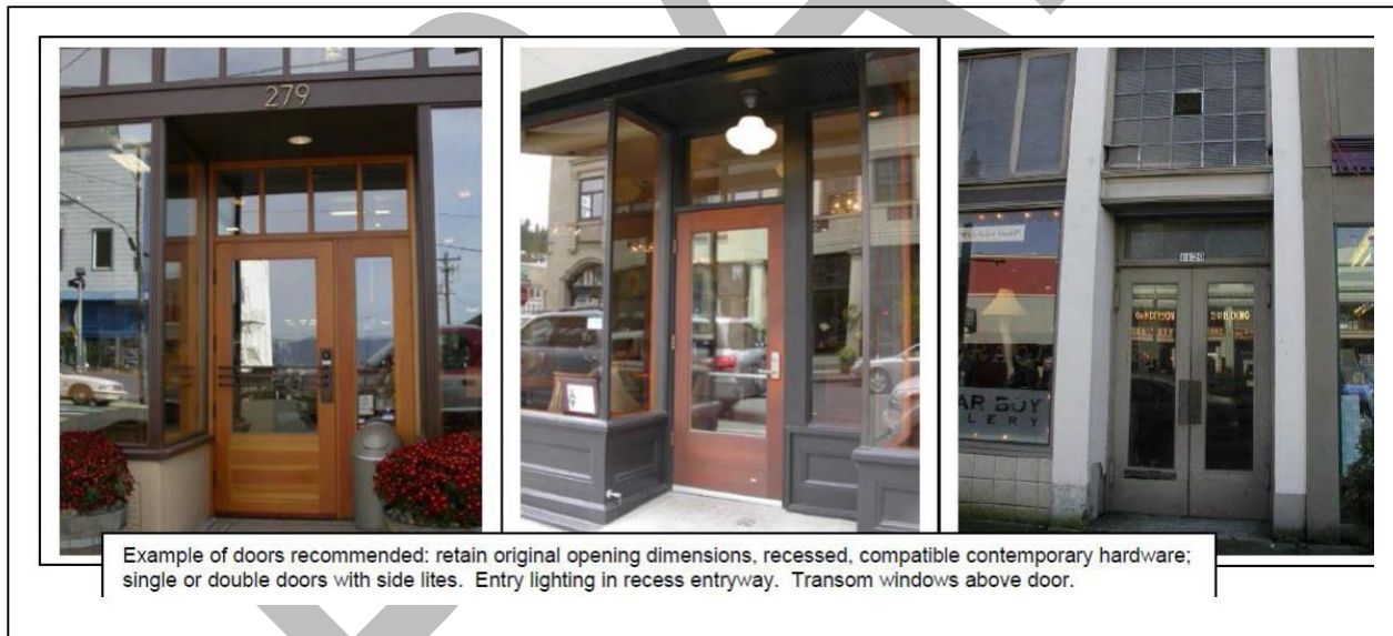
Figure 14.____- _: Recessed Doors, Contemporary Door Hardware, Single/Double Doors, Side Lites, and Transom Windows
